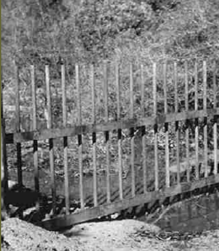
DEBRIS RACK (clearing sediment)
