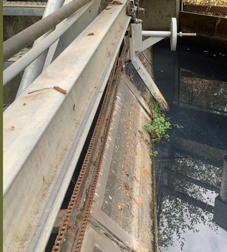
FISH SCREEN (screen fouling)
